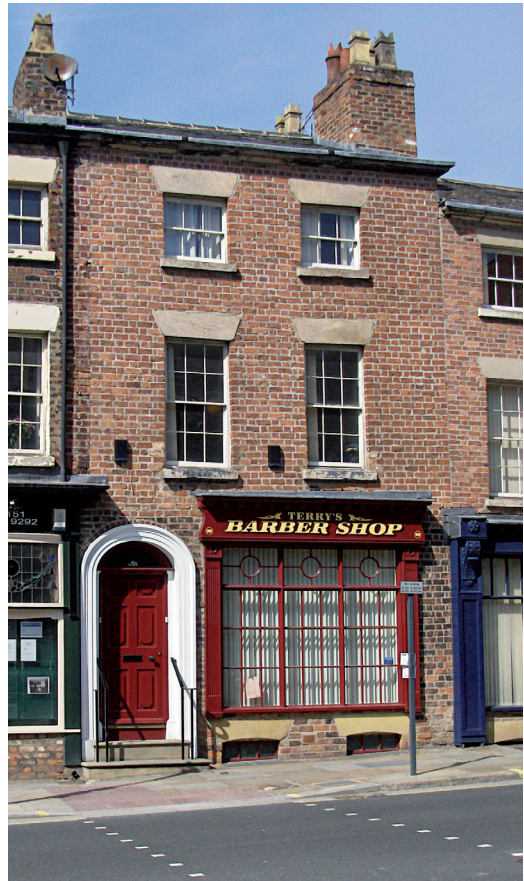
Fig. 9. 99 Mount Pleasant as it looks today. This was John Moncas' residence at the time of his bankruptcy. Little seems to have changed other than the road level and change of function from residential to commercial premises. Photo © Michael W. Paice.
